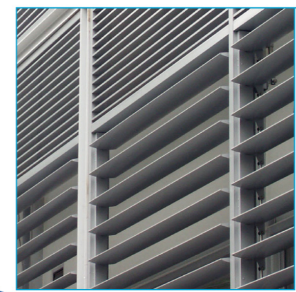
Linear actuator control Aerofoil movement Turn Angle : 110 degree
